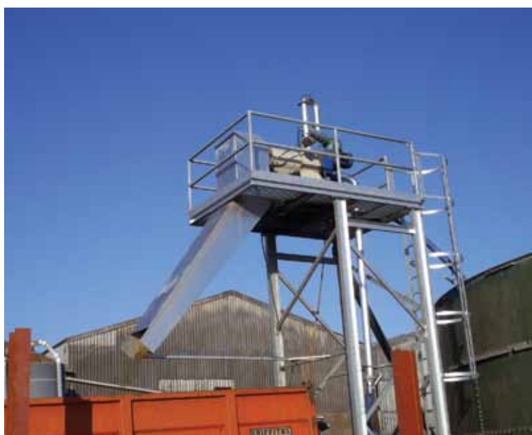
Separated solids being dropped into a trailer ready for transportation to an alternative site.
